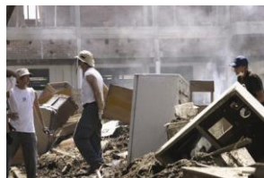
MR volunteers clearing the debris at the Muhammadiyah School.
