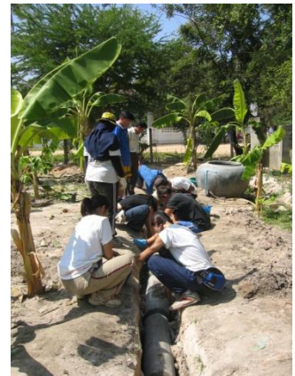
Drainage construction in Takeo, Cambodia.
