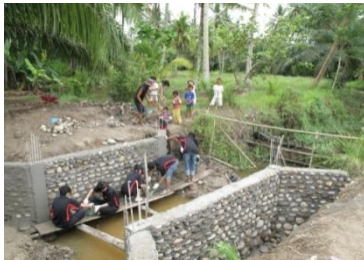
Singapore Poly MOVE team led by Deputy Director, Yuen Soo constructing a bridge at Hamparan Perak, North Sumatra, Indonesia.
